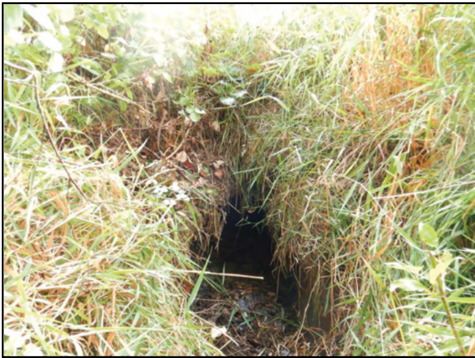
Figure 27. The old crossing was a 2.5 ft diameter concrete culvert.
