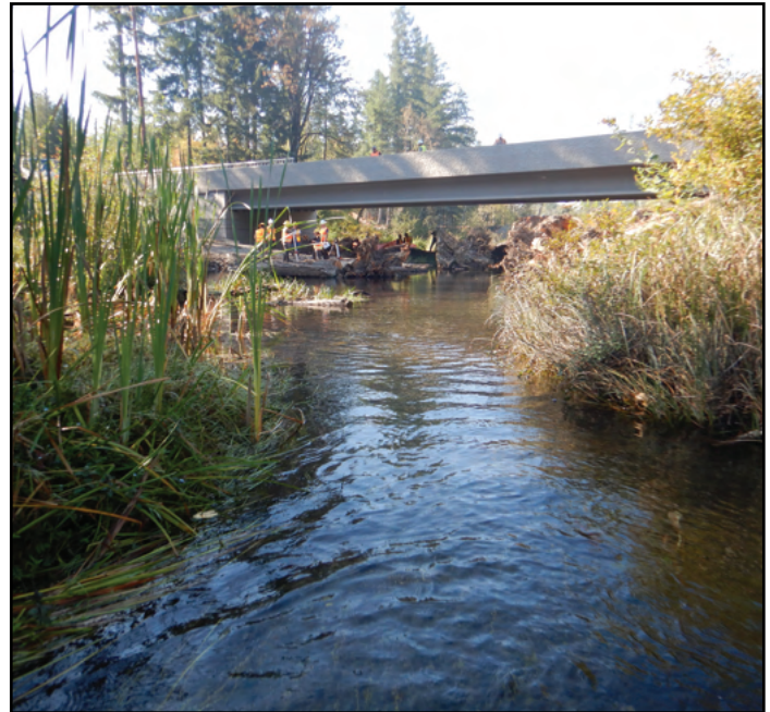
Figure 20. The new structure under SR 169 is a 113 ft long bridge. After construction, numerous juvenile salmonids were observed upstream of the project.
