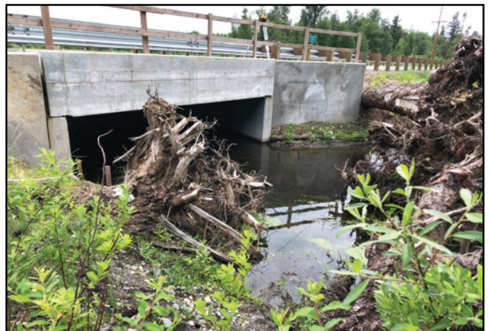
Figure 12. The new crossing is a 14 ft span by 8 ft rise concrete culvert.
