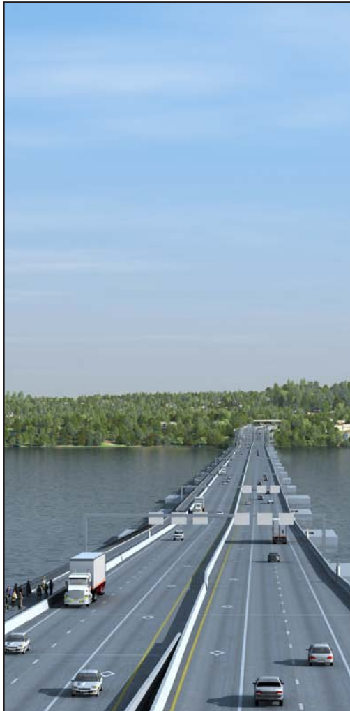
Conceptual rendering of the new SR 520 floating bridge that will include new transit/HOV lanes, a new bicycle/pedestrian path and shoulders.
