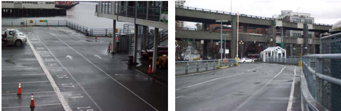
Exit Lanes at Seattle Ferry Terminal Exhibit 500-3
