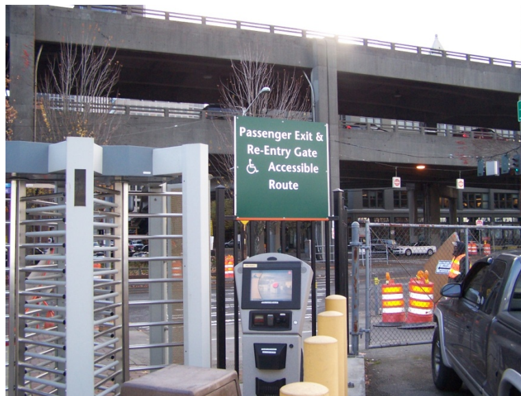
Pedestrian Gates at Seattle Ferry Terminal Exhibit 500-6
