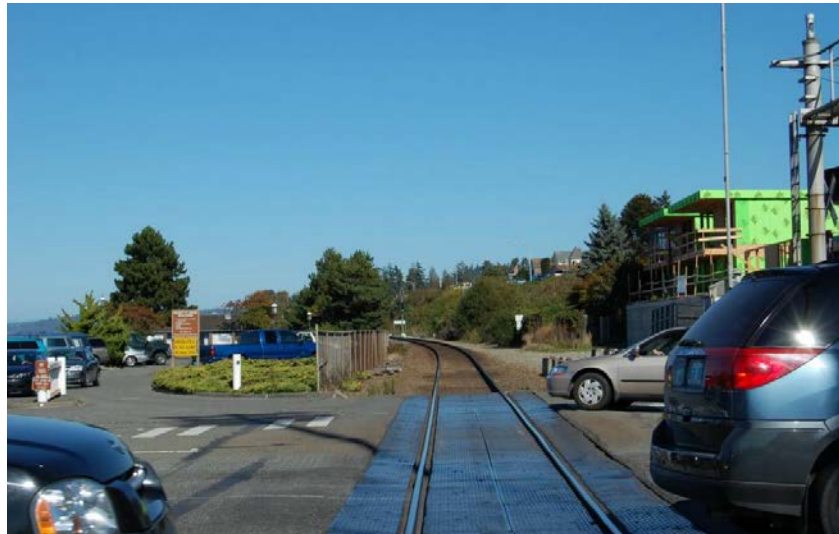
Railroad Crossing at Edmonds Terminal Exhibit 500-2
