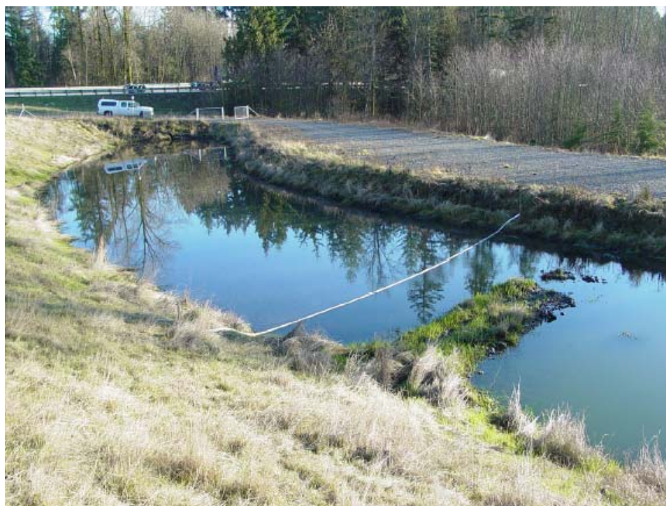
Oil Containment Boom Along I-5 in Thurston County.
