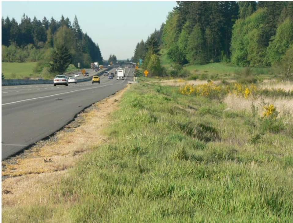
Engineered Dispersion Area Along I-5.
