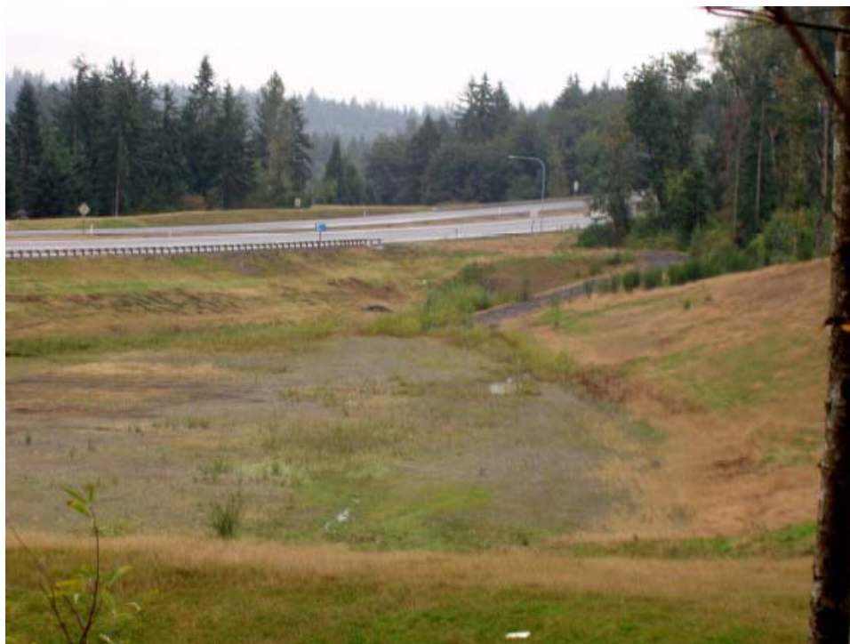
Detention Pond Along SR 18 in King County.
