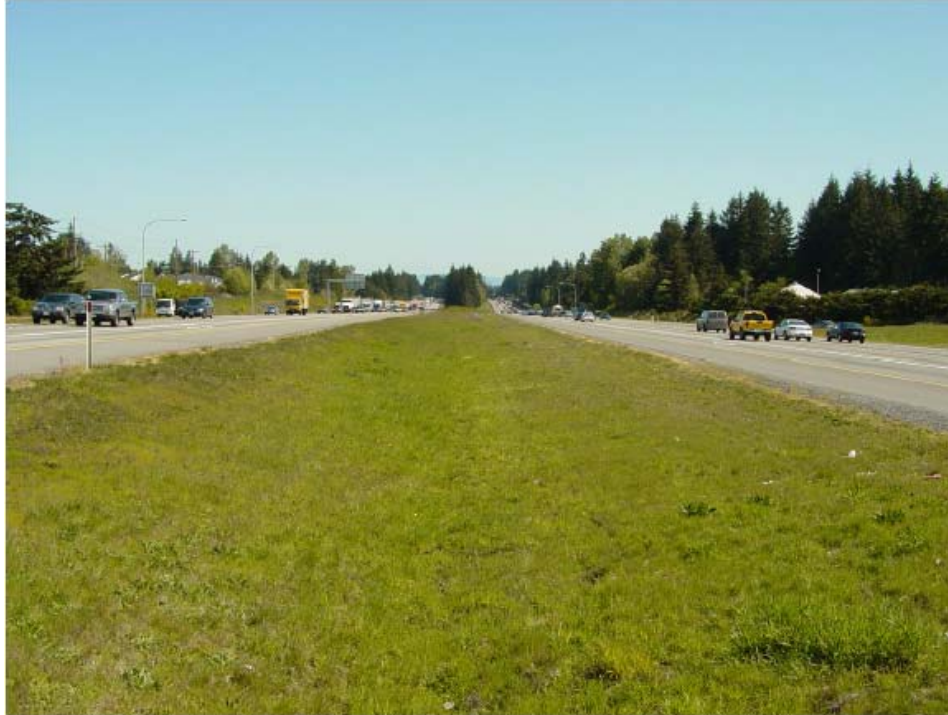
Vegetated Filter Strip in Median Along I-5 in Snohomish County.
