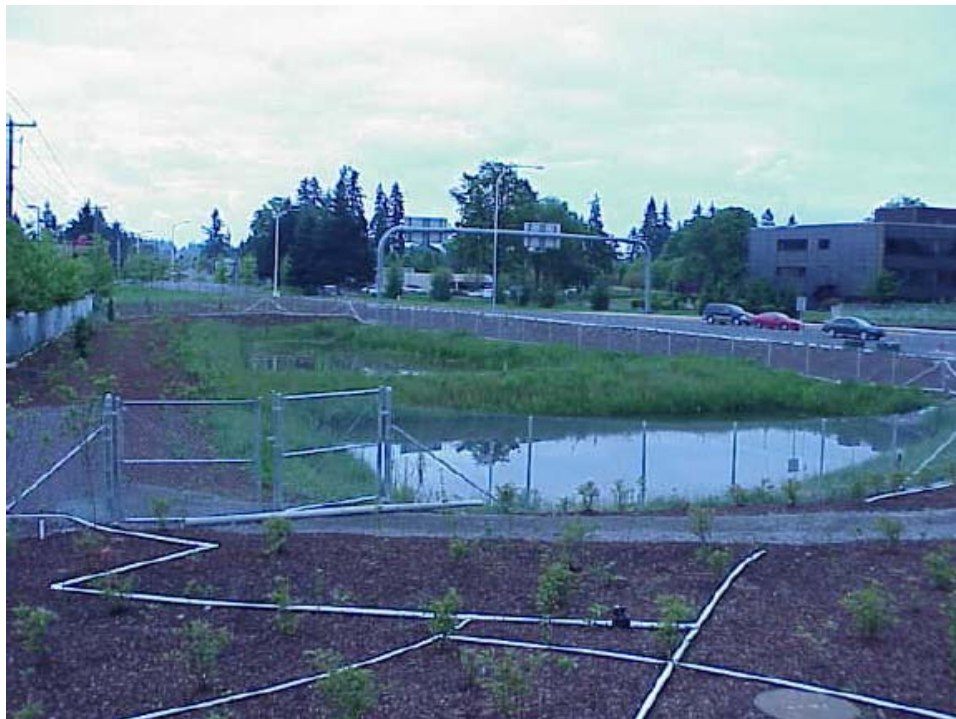
Combination Wet/Detention Pond Along SR 500 in Clark County.
