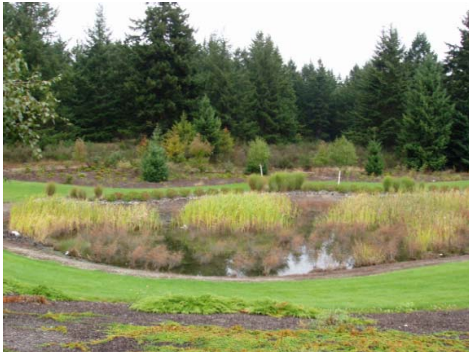
Infiltration Pond Along SR 510 in Thurston County.
