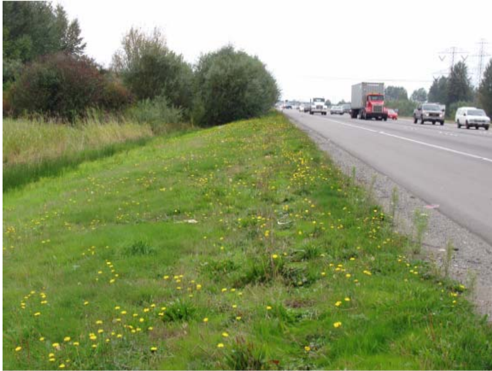
Ecology Embankment Along SR 167 in King County.
