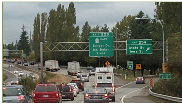
I-5 looking north between Lakeway and Iowa Street.
