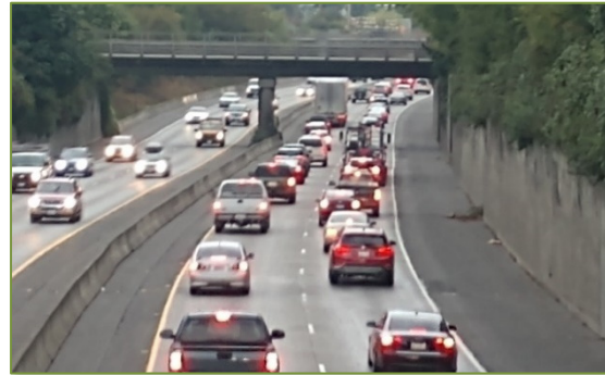
I-5 looking south from the Railroad Trail Bridge.
