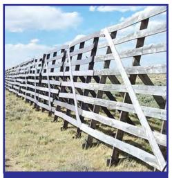
Permanent snow fences stop drifting snow from piling up on the highway. Placing a snow fence requires an understanding of snow drifting patterns, snow density, terrain, snow storage capacity, meteorology data, fence setback and drainage requirements.
