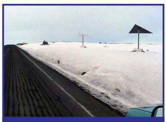
Pivoting in the wind, vortex generators redirect the natural airflow to clear the highway of snow on State Route 172, near Mansfield.
