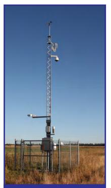
WSDOT has invested in advanced technologies designed to monitor, report and forecast road related weather conditions through the use of Road Weather Information Systems (RWIS).
