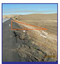
Example of where flattening to a 1V:4H or flatter would provide a reasonable side slope
