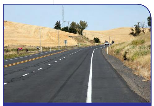
Passing lanes are often constructed on two-lane roadways to improve overall traffic operations by breaking up traffic platoons and reduce delays caused by inadequate passing opportunities over substantial lengths of roadway. The study extended from the junction of SR 27 just south of Pullman, to the beginning of the four-lane section just north of Spangle, MP 19.9 to 81.1. See Exhibit Geometrics - 2.
