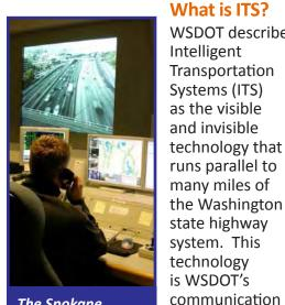
The Spokane Regional **Transportation** Management Center (SRTMC) is staffed 24/7 to monitor the areater Spokane roadways via traffic detectors and cameras, incident response coordination and providing upto-the-minute, weather, incidents, construction, and travel time information.
