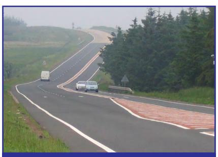
This 2+1 passing design configuration has a continuous three-lane cross section with alternating passing lanes.
