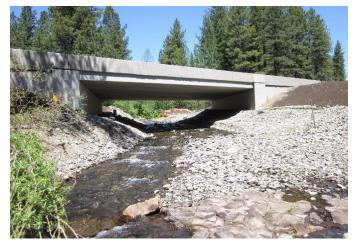
Figure 1. Fish and Wildlife Crossing Structure on U.S. 97 - a Fish Barrier Removal project that received terrestrial habitat connectivity enhancements.
